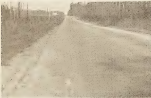
FIGURE 6.—APPEARANCE OF EXPERIMENT 7-B AT STATION 898 SEVEN YEARS AFTER CONSTRUCTION AND 3 YEARS AFTER THE ONLY SURFACE TREATMENT IT HAS RECEIVED.
